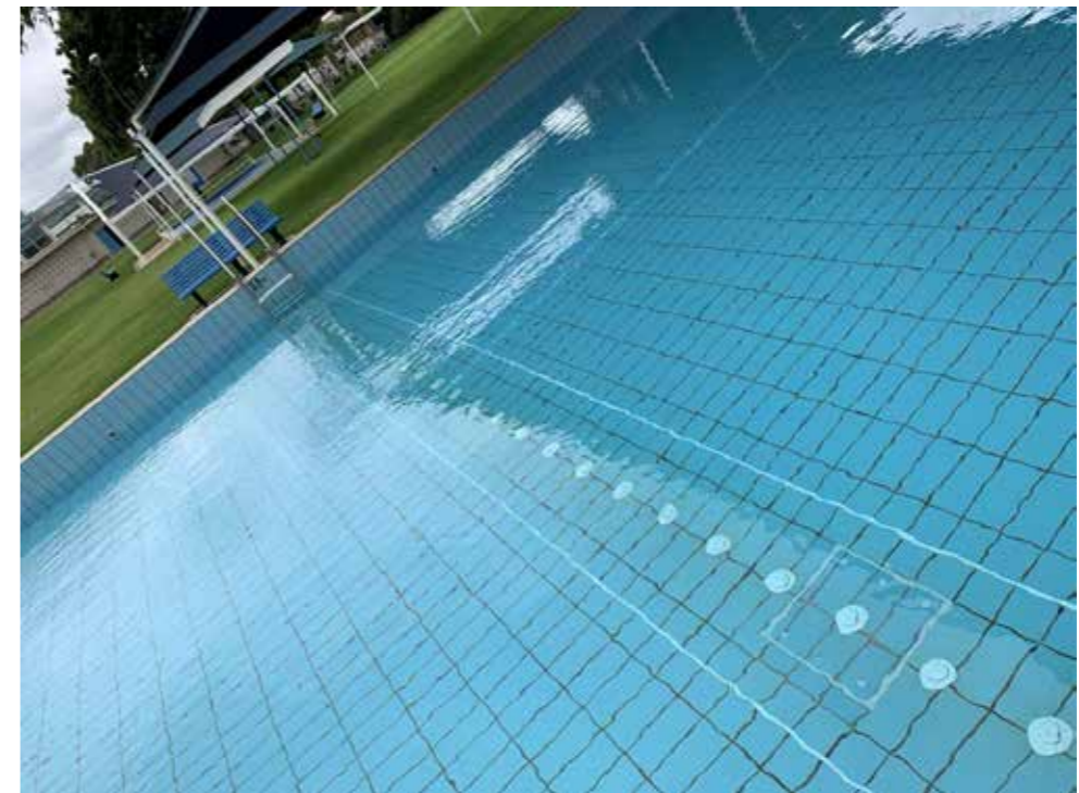
Figure 10: Floor returns in pool
