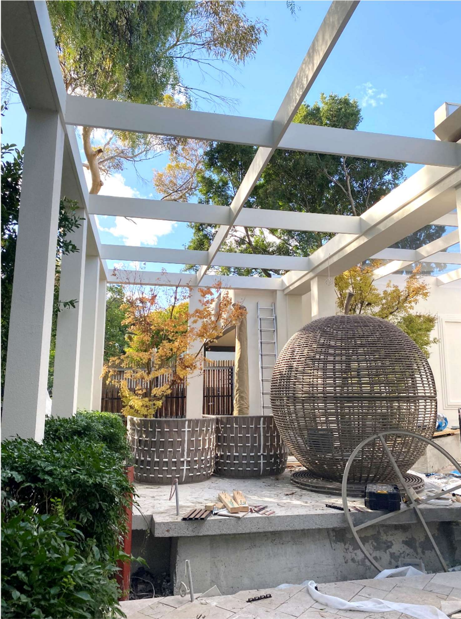
Photograph 2. Rear Pergola Extension
