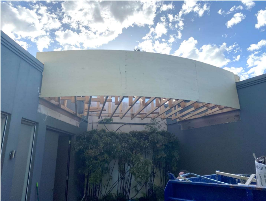
Photograph 1. Front Entry Roof
