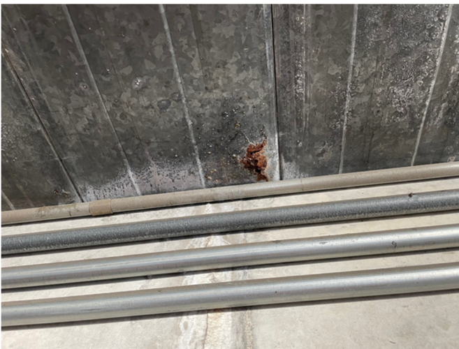
Figure 1 Rusted Bondek
