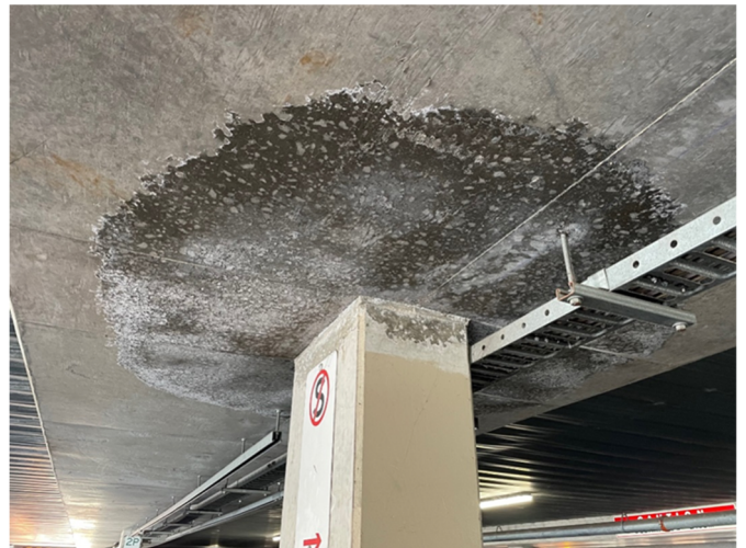
Figure 2 General efflorescence
