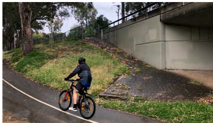
10. LINEAR PATH UNDER OBAHN OVERPASS
