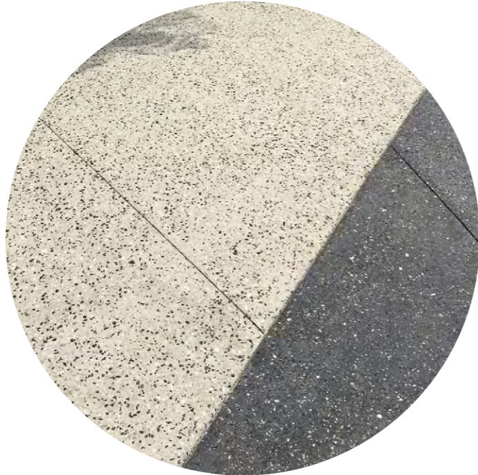
insitu concrete pavement
