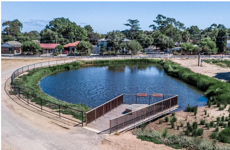
Felixstow Reserve Treatment Facility
